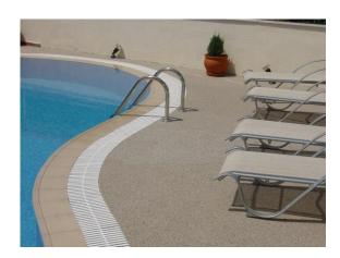
Consists of hard quartz aggregates and two-component polyurethane or epoxy resins. Grain thickness 0,7-1,2mm, 2-4mm and 4-6mm or bigger. For interior surfaces it is recommended the use of epoxy-based MARMOR STONE CARPET. Recommended for hotels, shopping centers, swimming pool surroundings, city squares and generally areas where high mechanical resistance and aesthetics are required.
