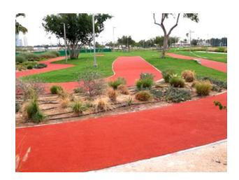
Elastic, seamless, flexible coloured flooring, ideal for jogging tracks in total thickness of 18mm.
