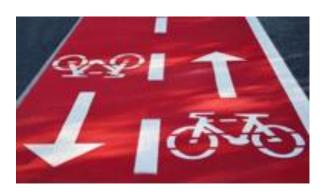
Consists of colored quartz aggreagates broadcasting (in granulometry of 0.7 mm - 1.2 mm) and two-component polyurethane resins for outdoor applications.
