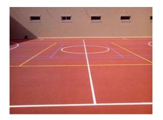
Very elastic shock-absorbent, cushion, wet-pour rubber flooring used as subfloor before exterior acrylic coatings and polyurethane coatings and as competitive sports courts system in combination with UV resistant top coating POLYSPORT XP 1069.
